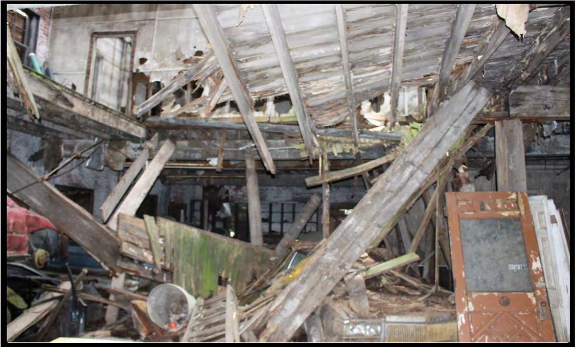
3 The first building is partially collapsed, and no hazardous materials were observed.
